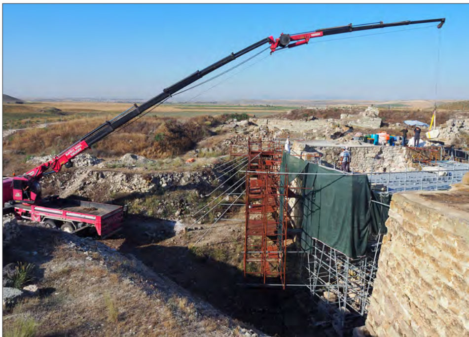
Figure 3: The crane lifting the restored blocks of the Early Phrygian East Gate from the scaffolding to their original position. Photo by Gebhard Bieg.
