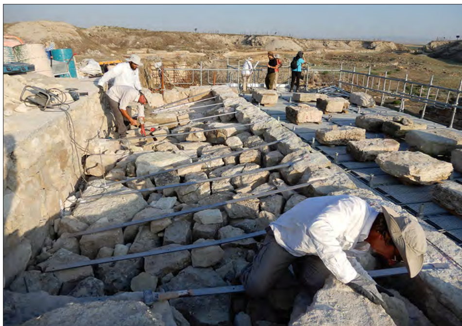
Figure 4: Installing the stainless-steel straps that anchor the facing stones of the Early Phrygian East Gate to the core of the wall. Photo by Gebhard Bieg.
