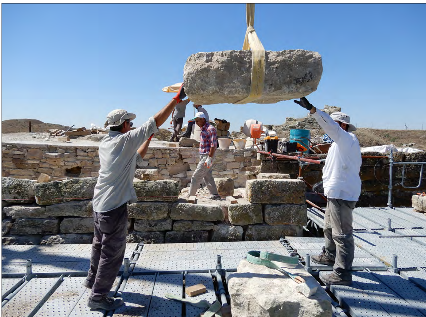
Figure 1: Moving the conserved stones of the Early Phrygian East Gate (9th c. B.C.) back to their original position. Photo by Brian Rose.
