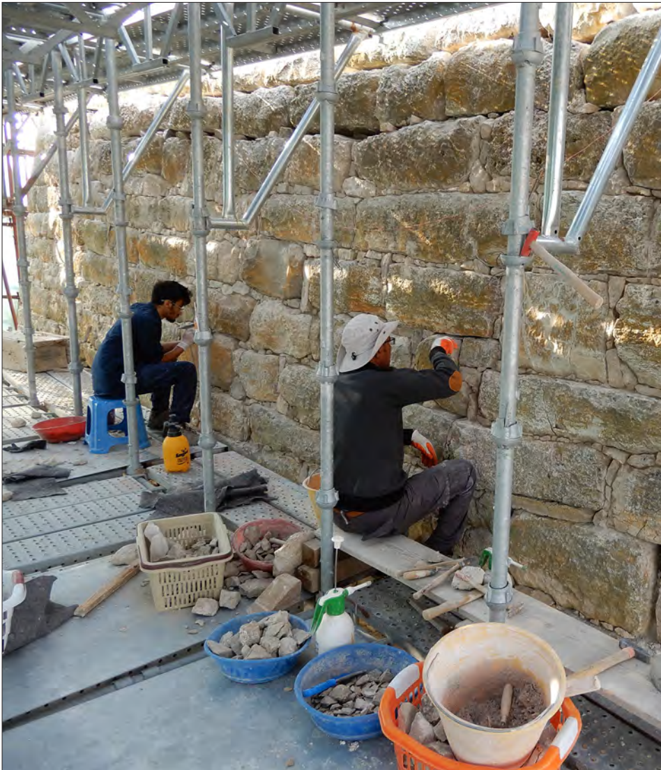
Figure 5: Repointing the wall face of the Early Phrygian East Gate's South Bastion. Photo by Brian Rose.
